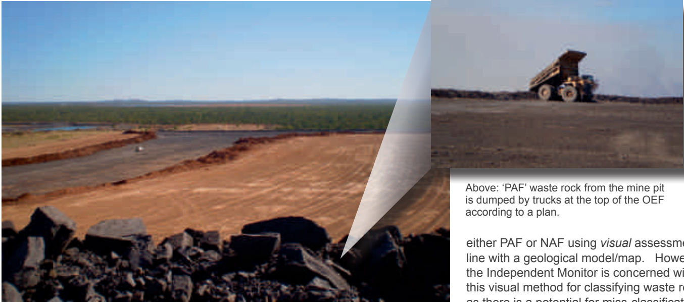
View from the top of the OEF looking at the clay base, with waste rock piled in the foreground.
